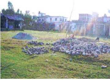
The site of the new Tikapur public library February 2007
